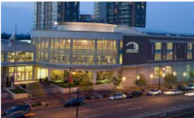
BU’s FitRec Center hosts many courts and recreational centers on campus. The Sustainability Revolving Loan Fund financed installation of energy-efficient light bulbs and occupancy sensors to reduce electricity use when the Center was unoccupied.
