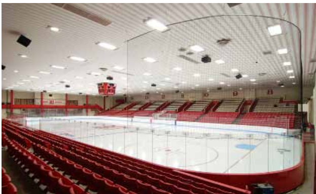
The Walter Brown Arena, located inside the Case Center, underwent lighting upgrades in the summer of 2010 that included occupancy sensors and installation of energy-efficient light bulbs.
